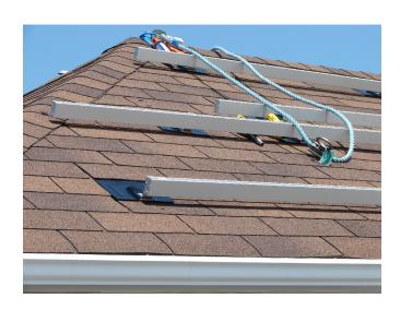
K-RACK™ is a complete solar panel racking system that is ideal for asphalt and steel pitched roofs, ground mounts, agricultural, commercial and industrial flat roofs. Our system can also be used to roof-mount satellite dishes and small antennas.
